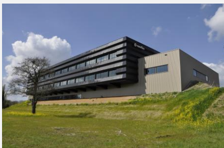
Environment Testing Amersfoort, The Netherlands 8,743 m 2
